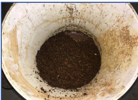
Rust Collected from the Existing Steel Chiller Lines
