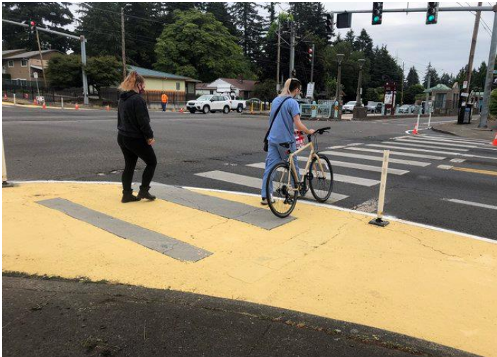
Temporary paint and barriers for intersection improvements
