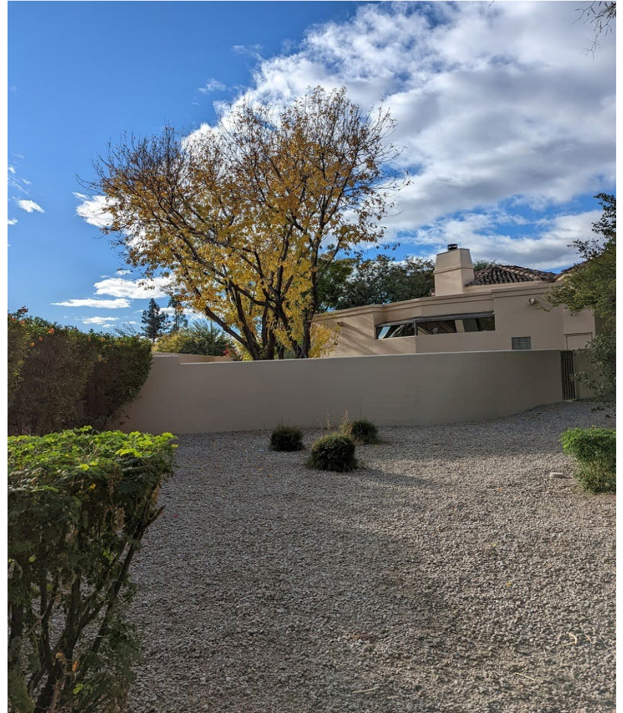
#2 Northeast Corner Facing South
