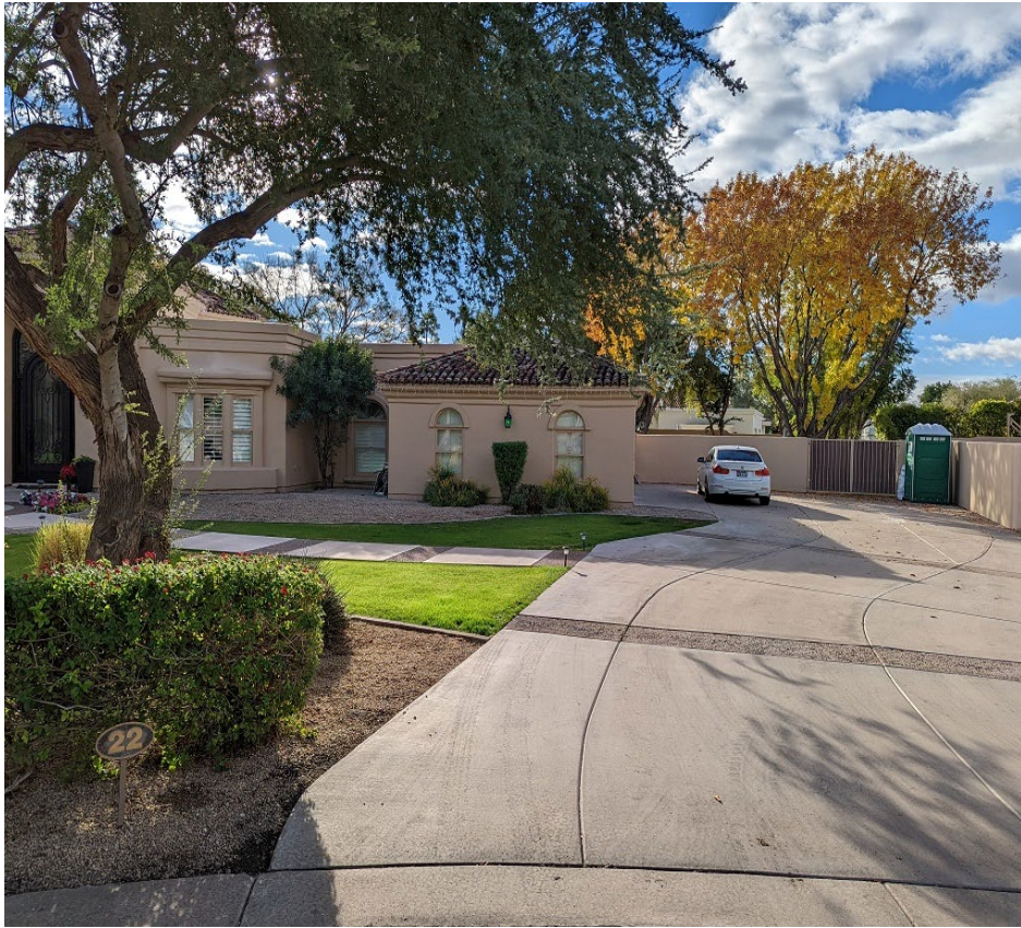
#1 Northwest Corner Facing South
