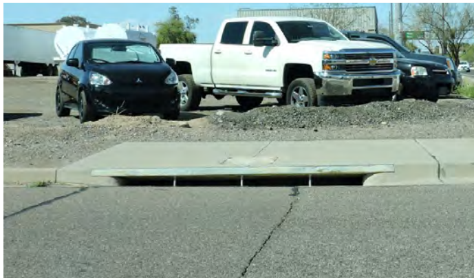
Figure 1. Typical Curb Opening Inlet Found at Siesta Lane and Rio Salado Parkway
