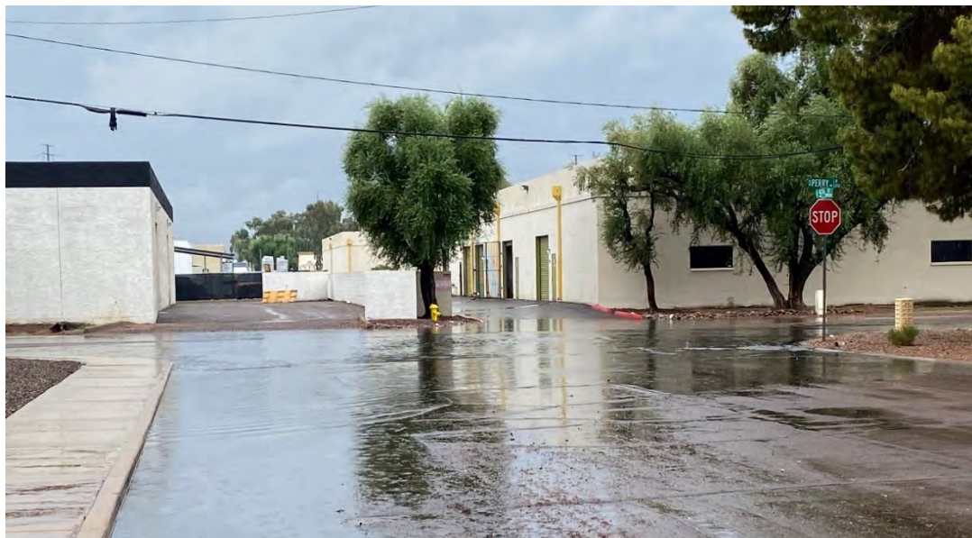
Figure 17. Street ponding on Perry Lane
