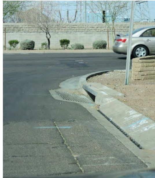
Figure 18. Stormwater inlets and slotted drains on Third Street at McClintock Drive
