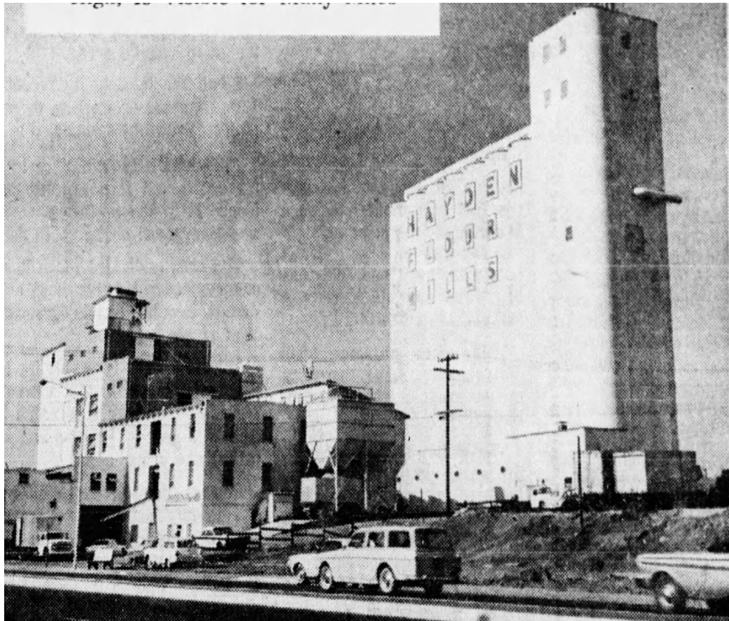
Figure 4. South and west elevations, view northeast, as pictured in 1966 (photograph by Mary Leonard, courtesy of Arizona Republic 07 August 1966: E1).
