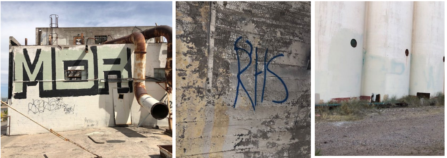
Figure 7. Examples of typical exterior paint and graffiti at the mill, including areas which have been vandalized and subsequently painted as an abatement strategy (Logan Simpson 2021).
