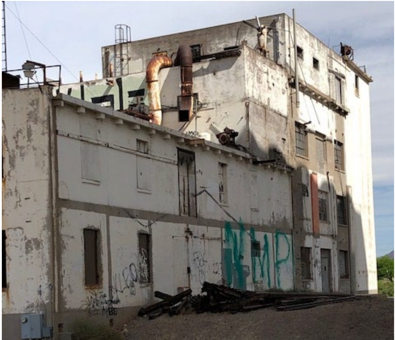
Figure 2. Photograph of exterior graffiti on the east elevation of the mill complex (Area 1). Photograph taken on April 16, 2021, facing northwest.
