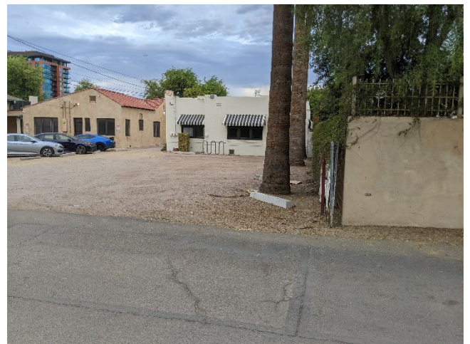
5. SW corner facing East
