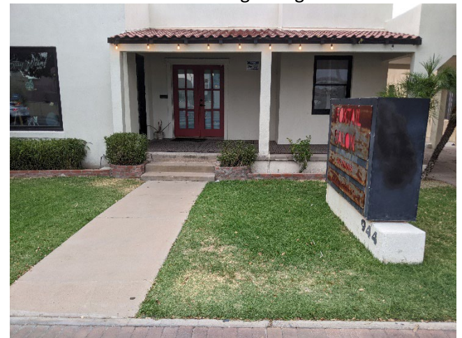
3. Front Entrance of building facing West
