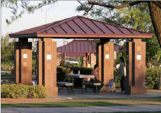
NOTCHED CMU BLOCK FINISH
