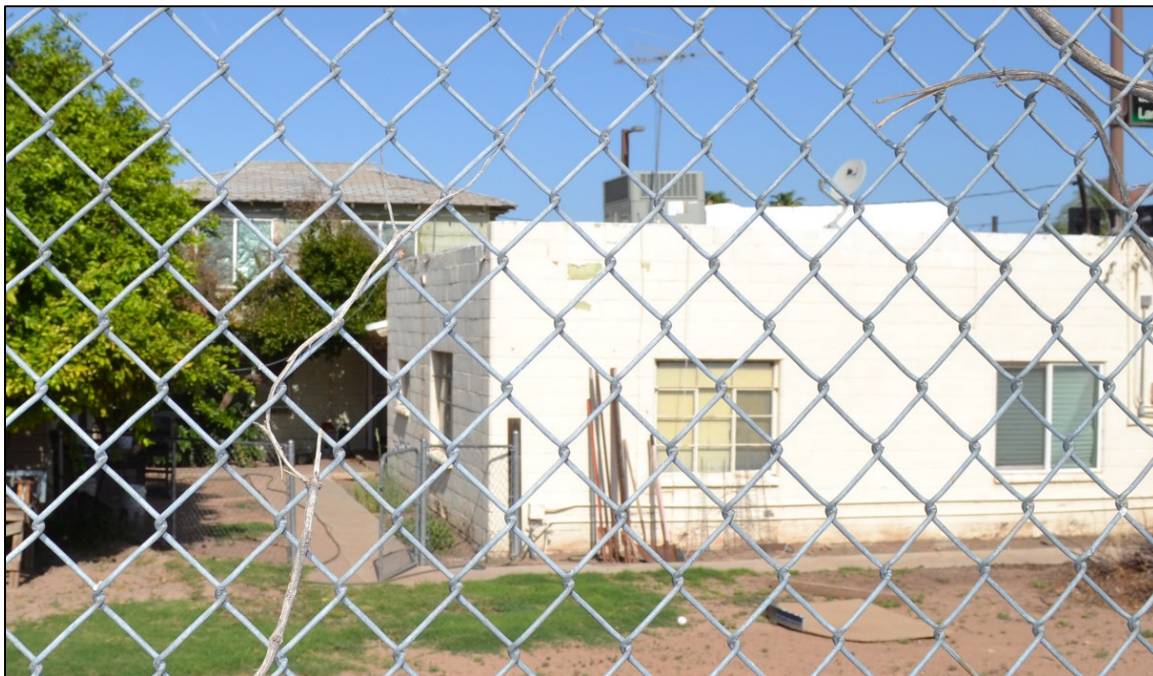
Figure 10. Overview of the Watson property with Building 1 in foreground (east addition), and Building 1a in the background (two story dutch-gable residence). view facing west.
