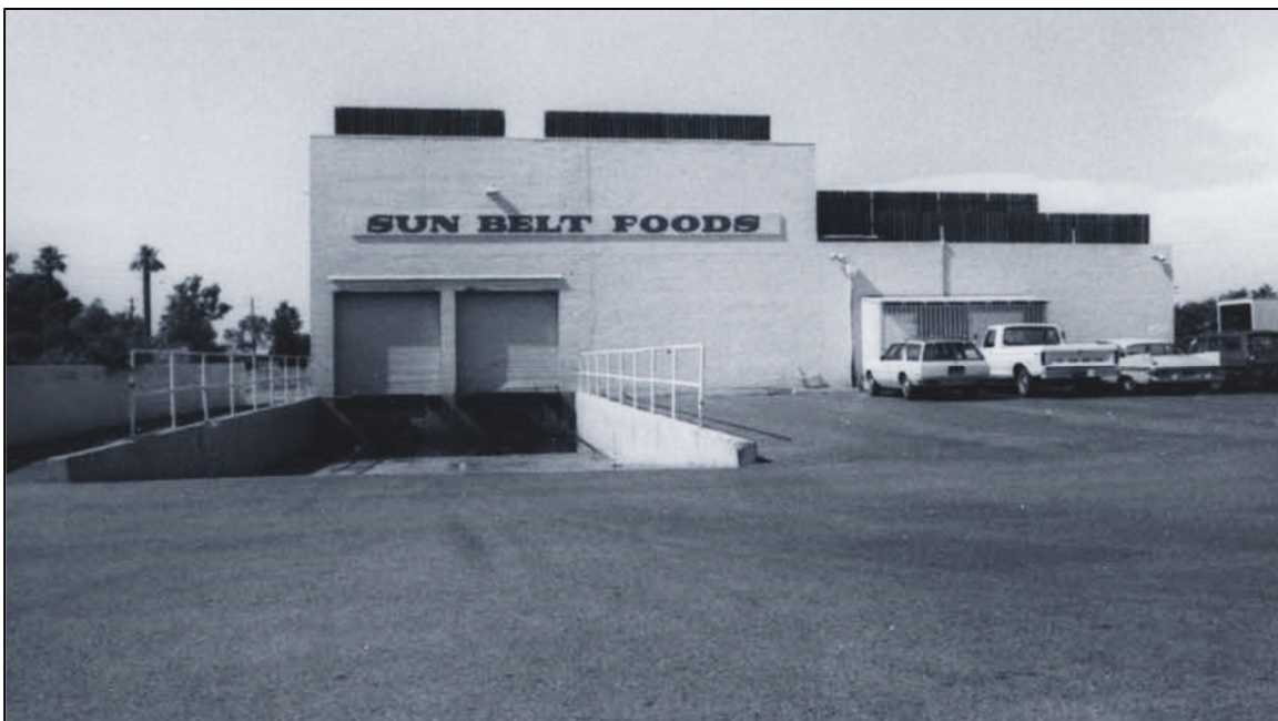
Figure 4. 1978 Overview of Building 2, view facing north. (THM Photograph Collection, Catalog No. 1992.2.137
