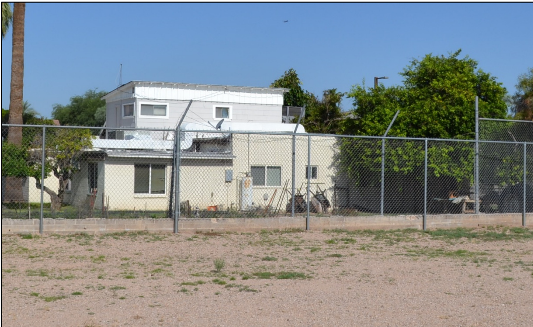
Figure 7. Building 1b, a single-story residence featuring a rear addition, as well as a side two-story addition with shed roof. View facing west from the South Apache Lot.
