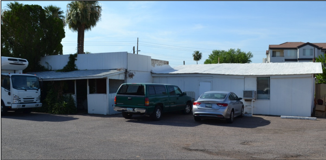
Figure 8. Overview of Building 1c, featuring a wood-framed west addition with a side gable roof (corrugated metal sheathing). View facing southeast.
