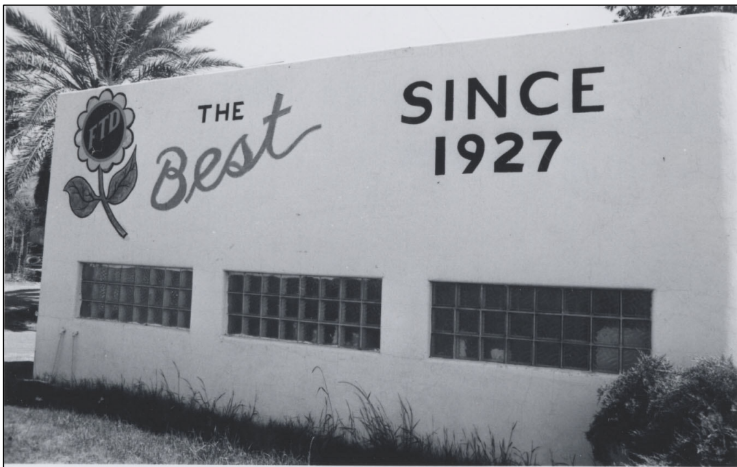
Figure 9. 1973 photograph of the eastern portion of Watson's Flowers, view facing southeast.
