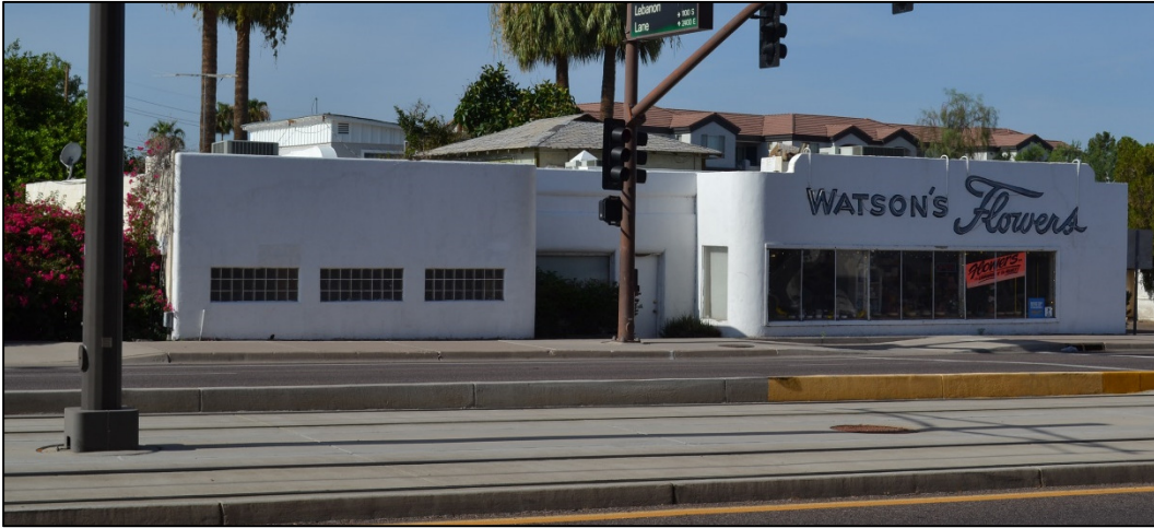
Figure 9. Front façade of Building 1, featuring the east volume (left), central portion, and west volume (right). View facing southwest.
