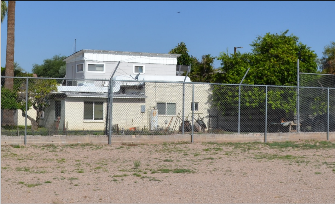
Figure 11. Building 1b, a single-story residence featuring a rear addition, as well as a side two-story addition with shed roof. View facing west from the South Apache Lot.
