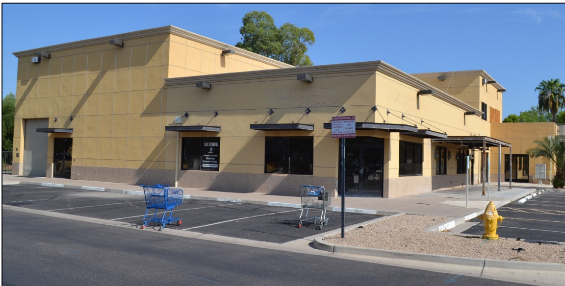
Figure 6. Contemporary overview of Building 2, view facing northwest.
