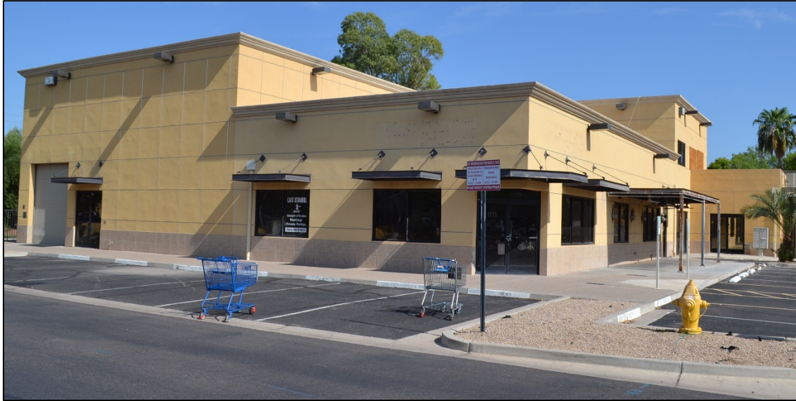
Figure 17. Contemporary overview of Building 2, view facing northwest.
