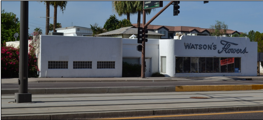
Figure 7. Front façade of Building 1, featuring the east volume (left), central portion, and west volume (right). View facing southwest.
