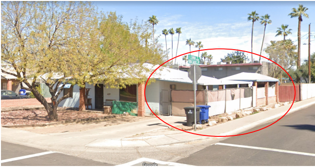
1029 S. BUTTE AVE Carport Addition within Street Side Setback
