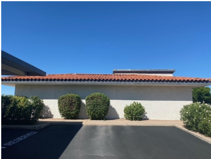
3. East side looking west
