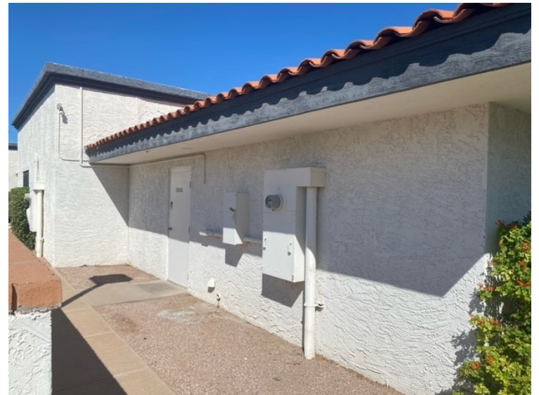
4. South side, back door looking north
