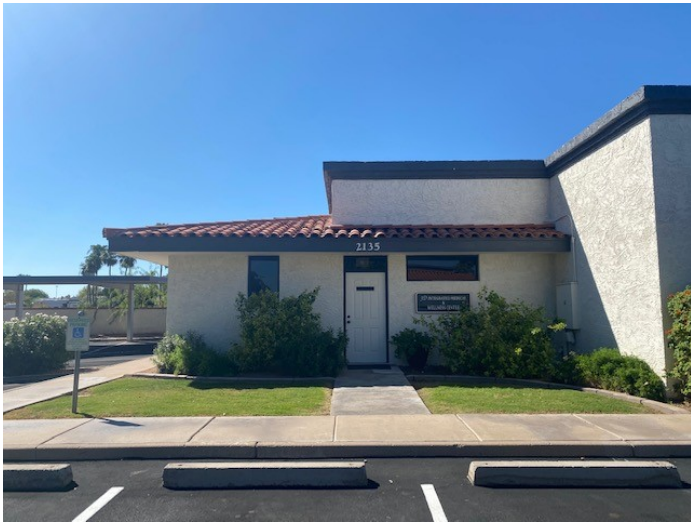
1. Front North Entrance looking south
