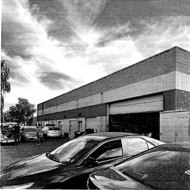
Photo #1: North elevation taken from the NW property corner facing eastward.
