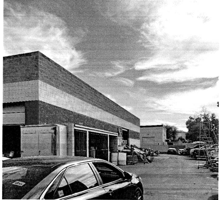
Photo #2: West elevation taken from the NW property Corner facing southward.
