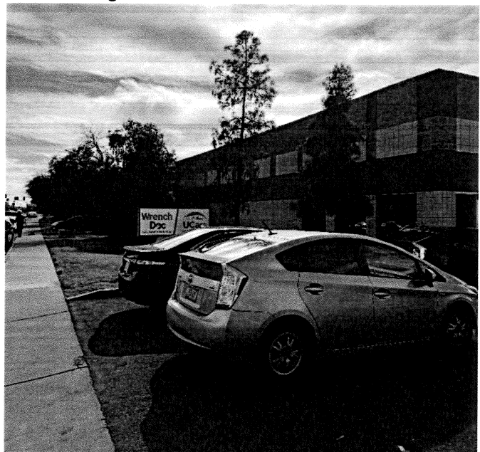
Photo #4: East Elevation taken from the NE property corner facing southward.
